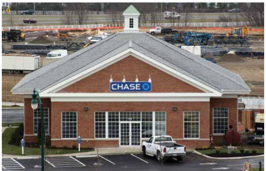
The 4,400-square-foot bank branch took 120 days from start to finish.
