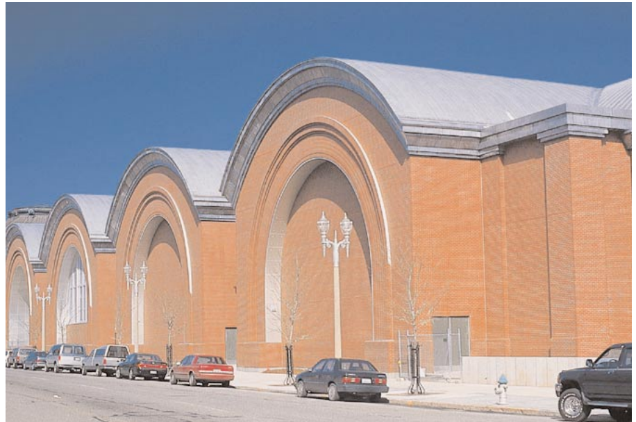
A series of eleven 55-foot-high reinforced concrete arches blend into the historic Union Station.
